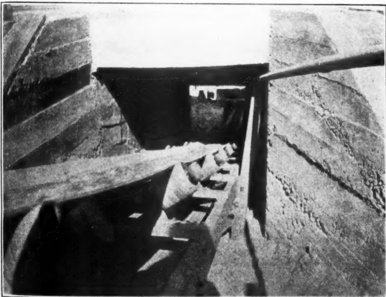
Tunnel Under Concrete Highway for Conveying Gravel to Bins
